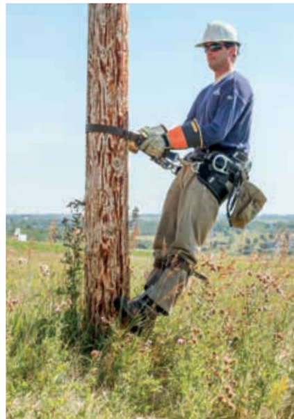
Years ago, linemen might have chosen to free-climb rather than use a positioning belt or “scare” strap. Now, OSHA requires linemen to use a fall-arrest device when climbing and working in the air, as demonstrated by Journeyman Lineman Seth Lothspeich .
